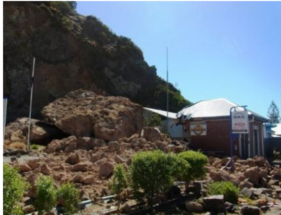
Figure 28. Huge rock fall adjacent to a building (Sumner).
