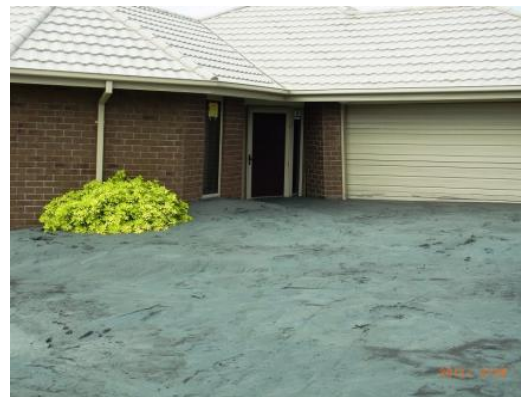
Figure 15. Damage to residential houses due to repeated liquefaction in Seabreeze Close, Bexley.
