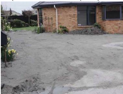
Figure 15. Damage to residential houses due to repeated liquefaction in Seabreeze Close, Bexley.
