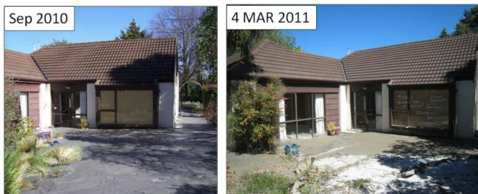
Figure 23. Repeated liquefaction in a residential property in North Kaiapoi.
