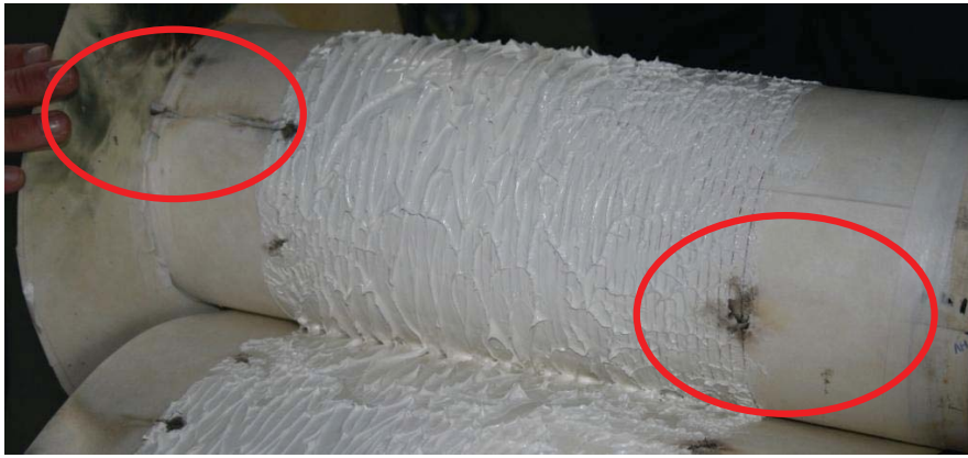
Figure 6 Flashover to the primary plasma short-circuited the secondary winding. Tracking is seen at the top and bottom of the winding, indicated by red circles.
