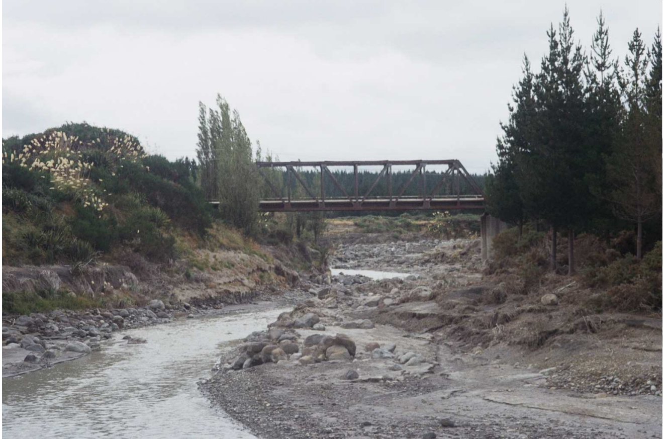
Figure 5 Whangaehu Rail Bridge March 2008, a year after the lahar.
