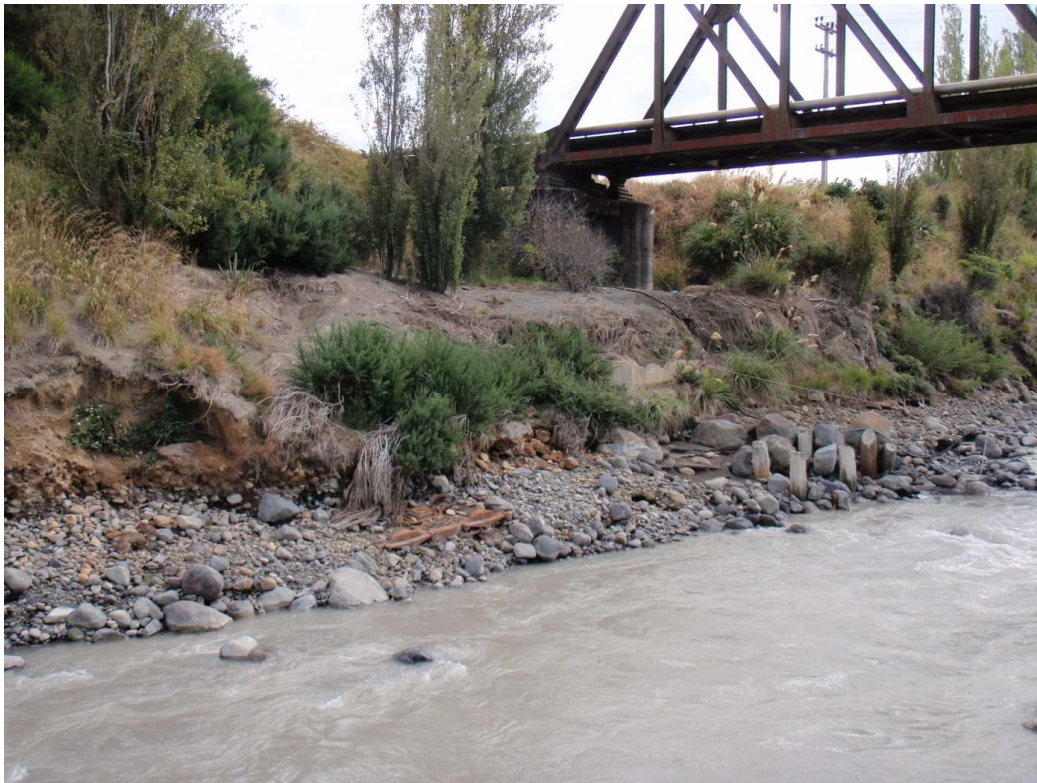
Figure 5 Undercarriage from the 1953 Tangiwai disaster exposed by the 2007 Lahar.
