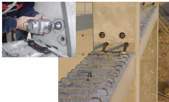
Fig. 11 – Prestressing the inclined bars
