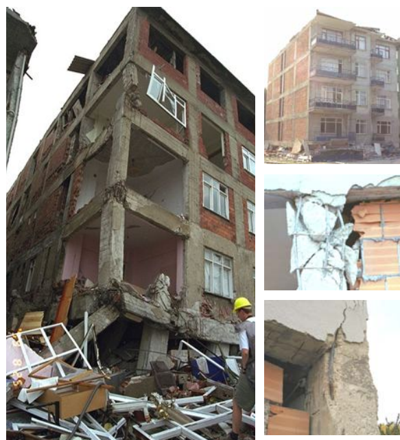
Figure 2. Observed global and local damage in under-designed existing R.C. frame buildings with infills (left and top right, Izmit-Kocaeli and Athens earthquakes in 1999, from NISEE Image Collection; centre and bottom right: Molise event 2002).
