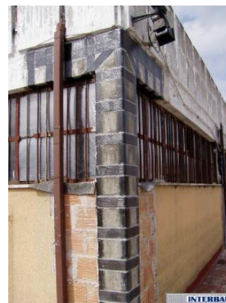
Figure 10. In situ FRP-retrofit of the exterior face of a corner beam-column joint
